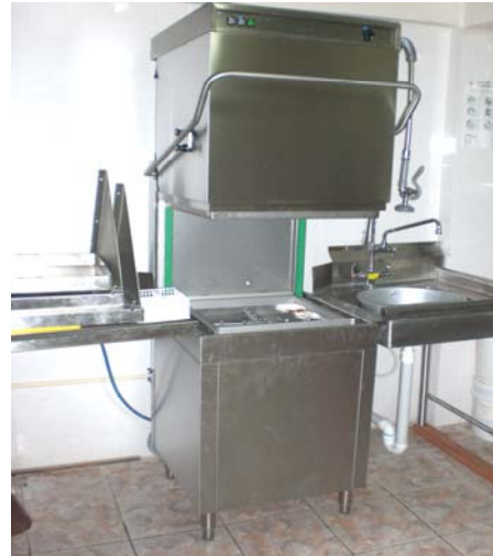
Newly installed commercial dishwasher
